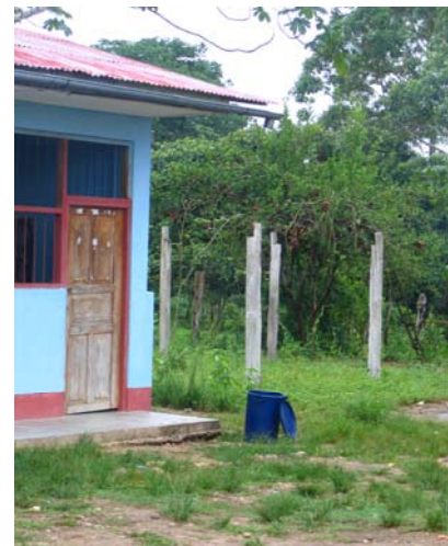
Above: Rainwater harvesting is not widely practiced in Curimaná. However, in this example where rainwater is collected from a painted roof, the collected water is likely contaminated with paint flakes.
