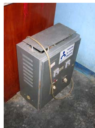
Above: The chlorine generator at the Curimana Health Post
